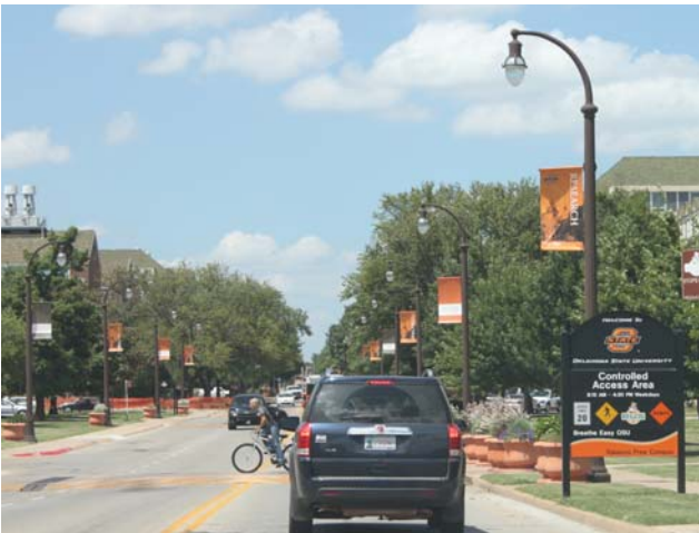
Monroe Street Lighting
