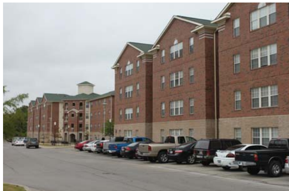
Cleveland Street (Currently a Parking Lot Aisle)
