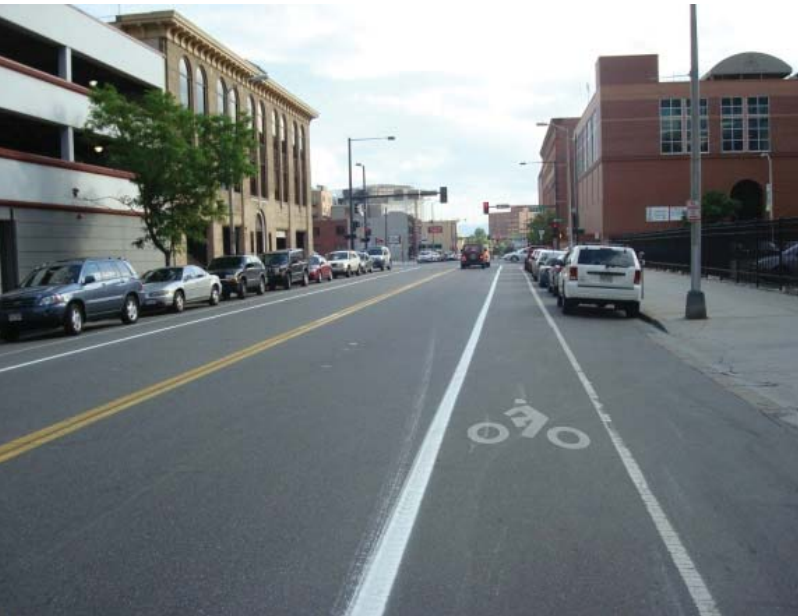
Example of a Class II Bicycle Facility
