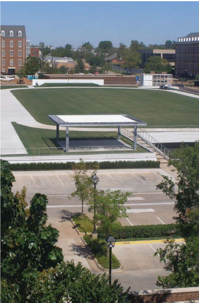
Chesapeake Central Car Park, Oklahoma City, OK - Airfield Systems® Airpave® porous paving system provides a durable / cool surface for festivals and recreation over a parking garage.
