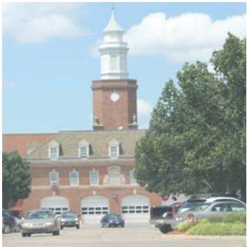
Campus Fire Station
