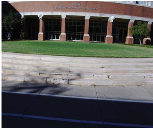
9. Advanced Technology Research Center Steps / Terrace Renovation
