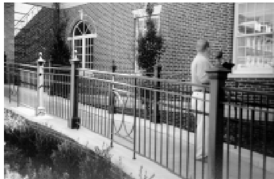
Railings Photograph C, Willard Hall.
