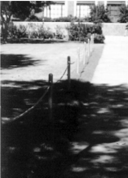
Railings Photograph G. Post and Chain Type to be Removed.
