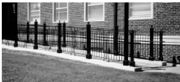
Railings Photograph A, Human Environmental Sciences Building.
