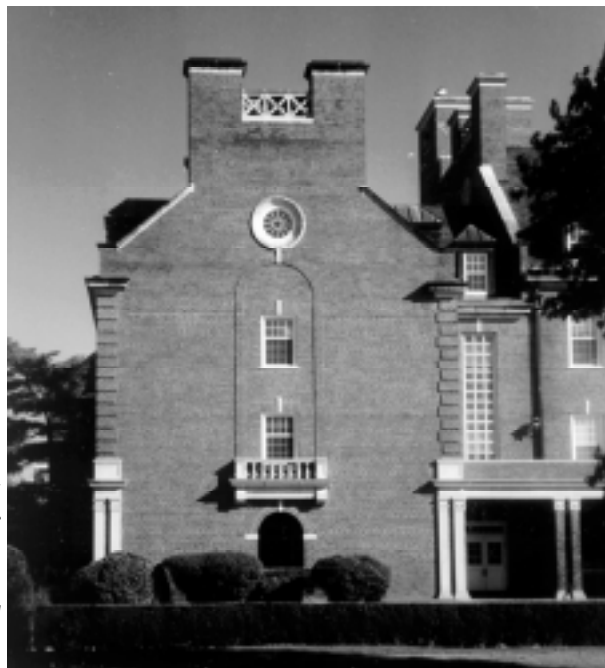
Wall / gable roof end at Student Union with double chimney components, ionic pilasters at building corners, double columns supporting a portico, brick quoin detailing of corner, double sash windows, small circular window, and balcony element with balustrade.
