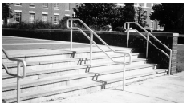
Railings Photograph B, Edmon Low Library.
