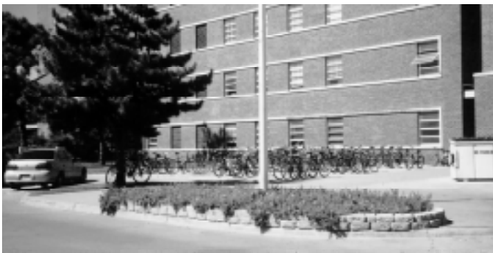
Wall Photograph H, Agricultural Hall.
