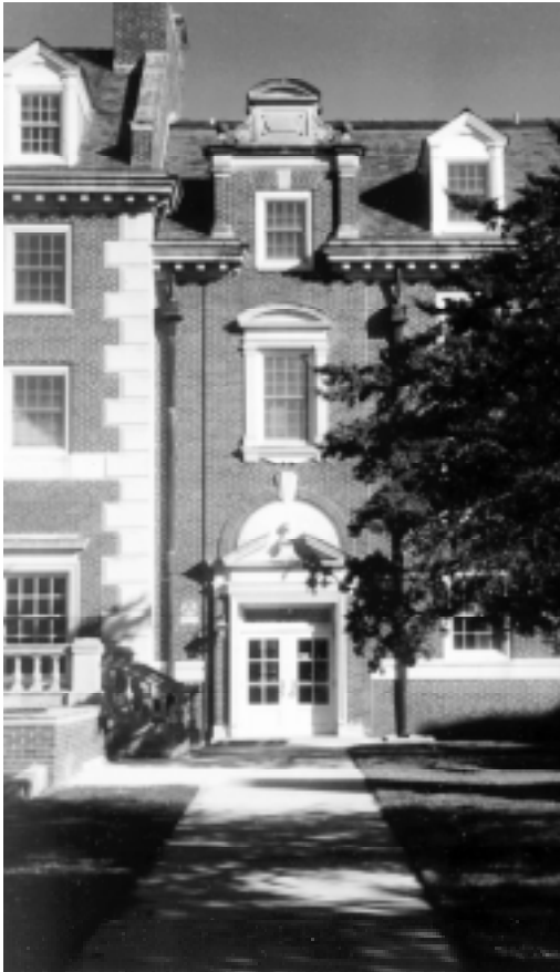
Entry at Cordell Hall with broken pediment above the doorway. The entry component is further expressed by a slight projection extending the entire height of the façade. Building corners are defined with cast stone quoins.
