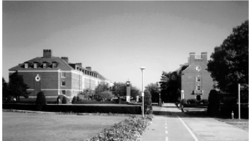
Variations in roof styles occur on campus, as illustrated in this photograph of the Student Union (right) with a gabled roof and the Classroom Building, which has a hip roof. Both styles occur in traditional Georgian architecture.
