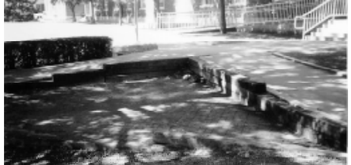
Wall Photograph E, Life Science East.
