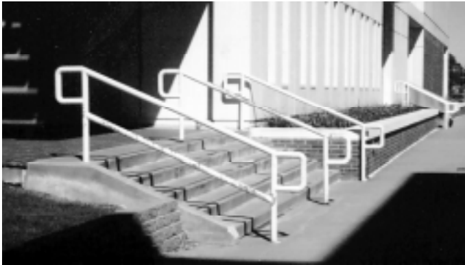
Railings Photograph J. All railings should be dark to minimize appearance, unlike this Railing at the Noble Center (Refer to Railings Requirements on previous page.)
