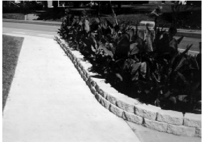
Wall Photograph G, Hester Street and University Avenue.
