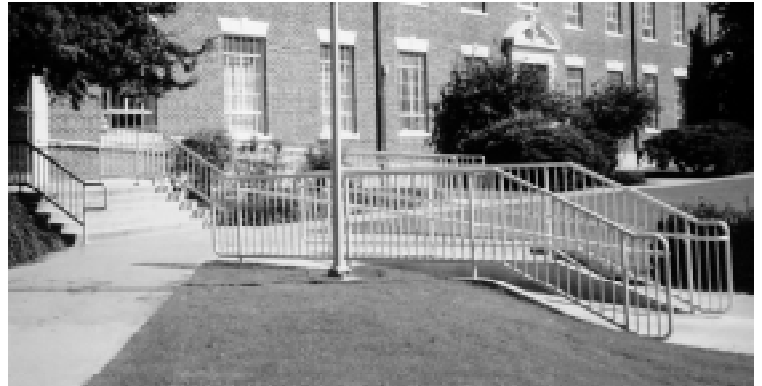
Railings Photograph K. Vertical Members in Railings on Grade Should Be Minimized to Simplify Appearance, unlike this Existing Railing.
