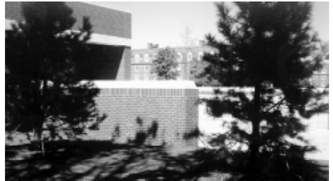
Wall Photograph C, Advanced Technology Research Center.
