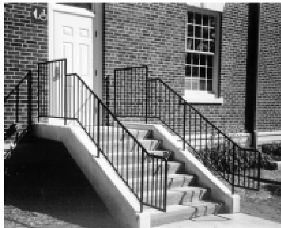
Railings Photograph F, West Side, Willard Hall.
