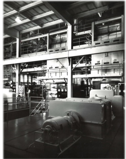
Figure 1, Existing Power Plant
