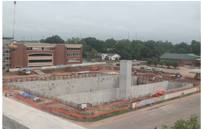
Figure 48, Central Plant Construction Progress, as of 6/13/2016
