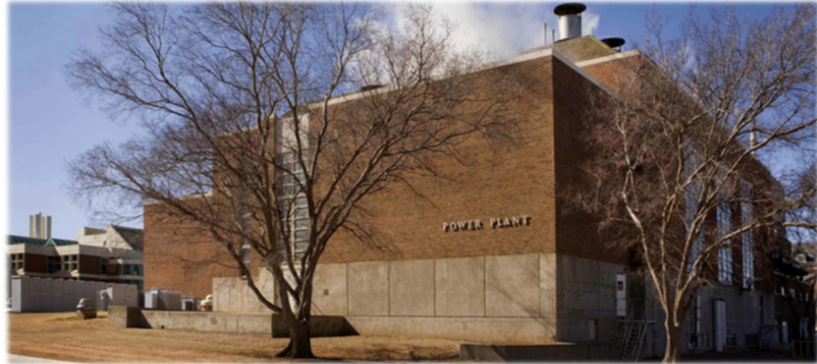
Figure 11, Existing Power Plant – Constructed 1947
