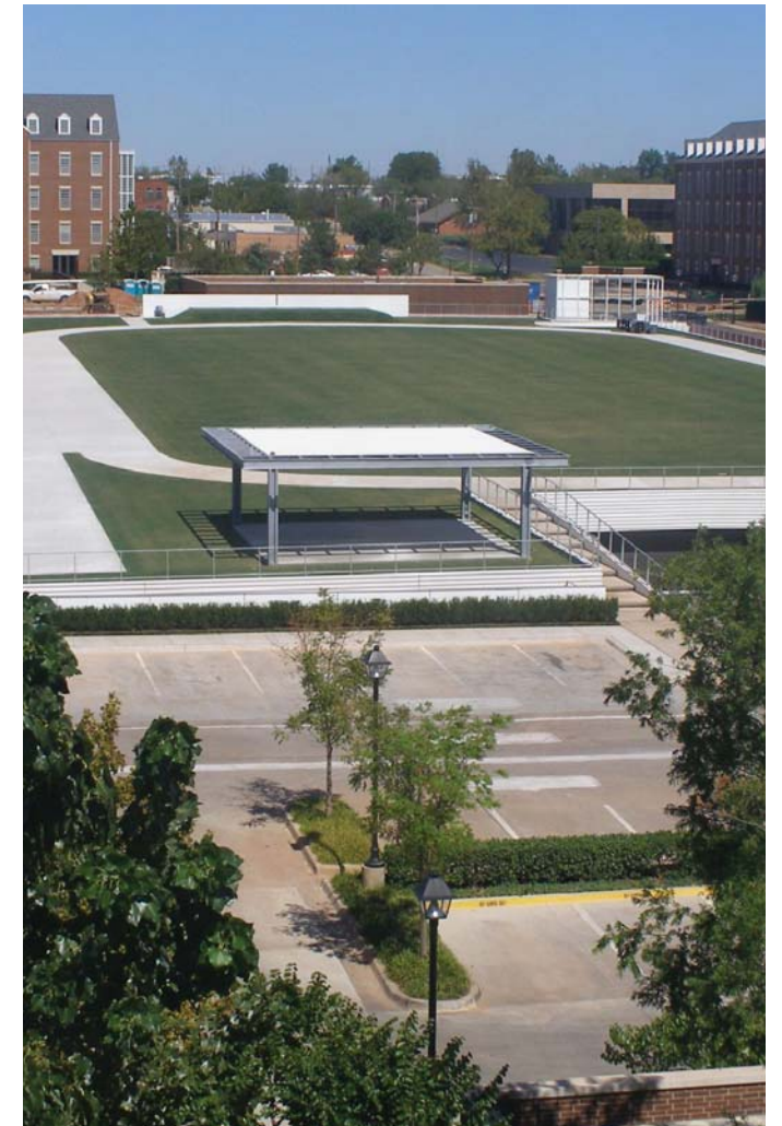
Chesapeake Central Car Park, Oklahoma City, OK - Airfield Systems® Airpave® porous paving system provides a durable / cool surface for festivals and recreation over a parking garage.
