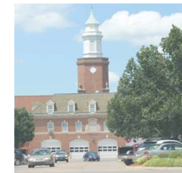
Campus Fire Station
