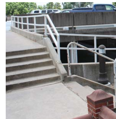
Student Union Parking Garage
