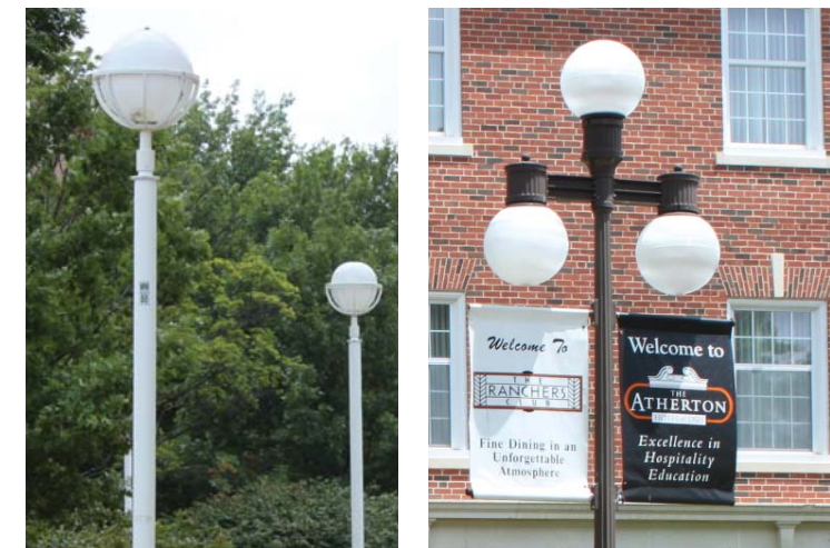
Globe Style Light Fixtures near the ATRC (left) and Atherton Hotel
