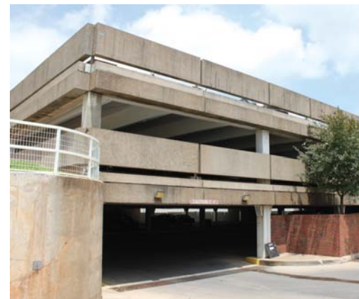
3. Student Union Parking Garage Facade
