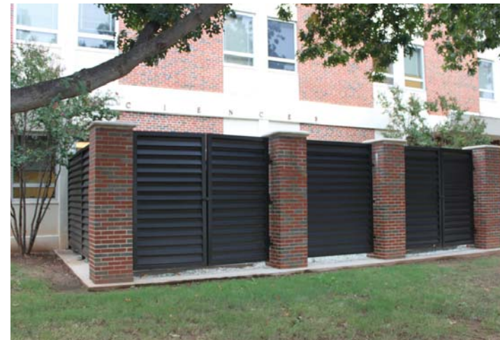
Good example of a screening enclosure at the Math Sciences Building shows 'OSU Blend' brick, cast stone caps and black metal doors
