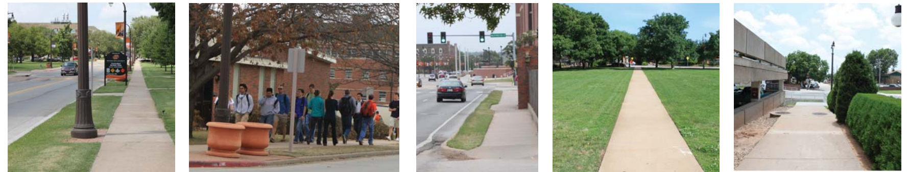
The majority of the campus is served by walkways that are too narrow. Prime examples are walks along Monroe Street (left) and walks along Hall of Fame Avenue (center).
