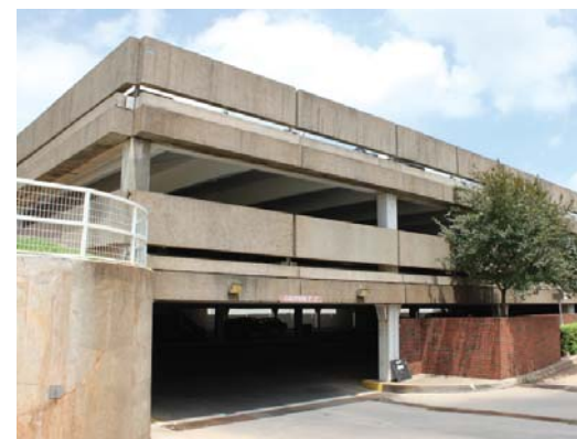
Student Union Parking Garage
