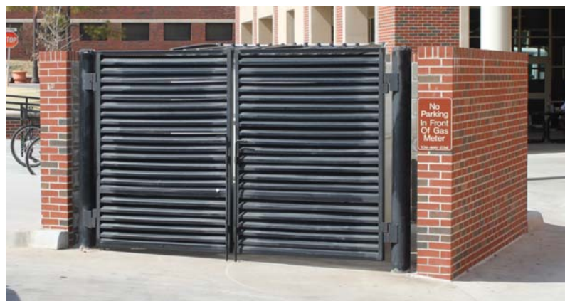
Good example of a dumpster enclosure at the N. Classroom Building shows 'OSU Blend' brick and black metal doors (should include a cast stone cap)
