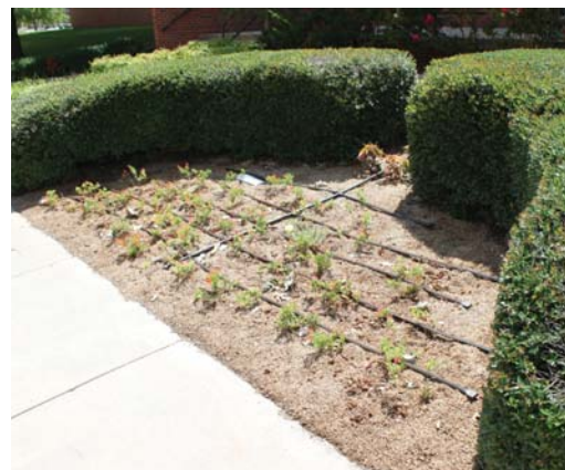
6. Ag Hall Main Entry Landscape Renovation
