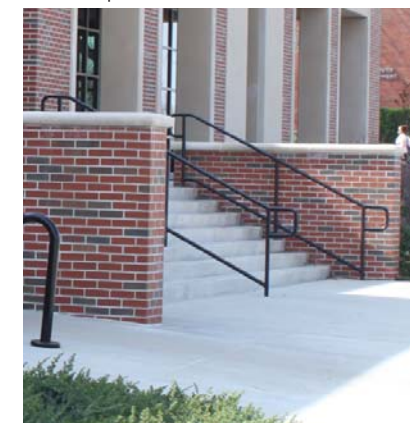
Good example of standard black handrails at the N. Classroom Building
