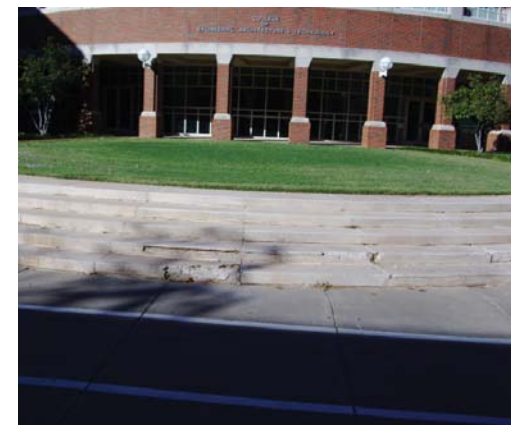
9. Advanced Technology Research Center Steps / Terrace Renovation
