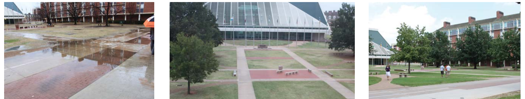
International Plaza is a very prominent space within the OSU campus, but at the present time is not a comfortable pedestrian space. As shown in the photo to the left, poor drainage is an issue on the International Plaza, as well as many other areas across the campus
