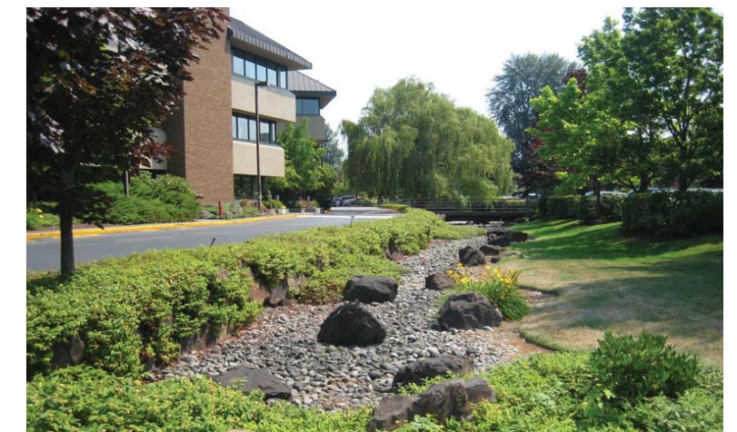
Proposed sustainability enhancements include diverse strategies such as drip irrigation, permeable paving systems, composting and bio-swales.
