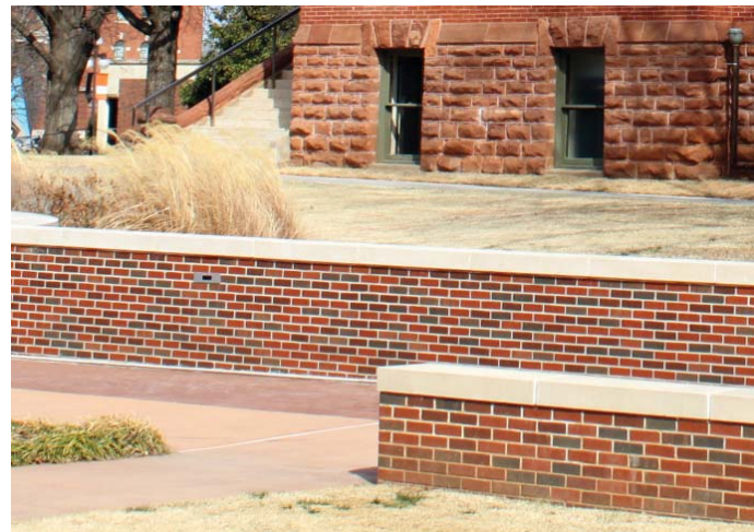
Good example of freestanding and retaining walls near Old Central shows standard 'OSU Blend' brick and cast stone wall caps
